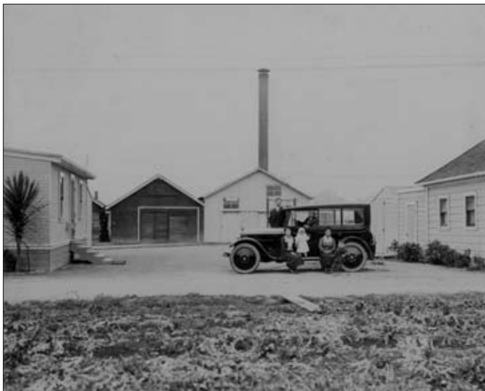
The Nabeta nursery at Potrero Avenue & 50th Street ca. 1923. On the running board: Takayo(m), Fumiko(d), Michiko(gm) & Toshiro(s). Behind them are Torataro(f) and Yataro(gf). From the left are the main house, shed, boiler house and housing for the hands. ECHS collection, courtesy of the Doi family.
